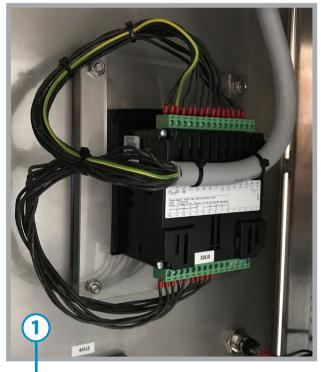
Programmable logic controller (PLC) With built-in high resolution, full-color touchscreen & onboard I/O configurations.
